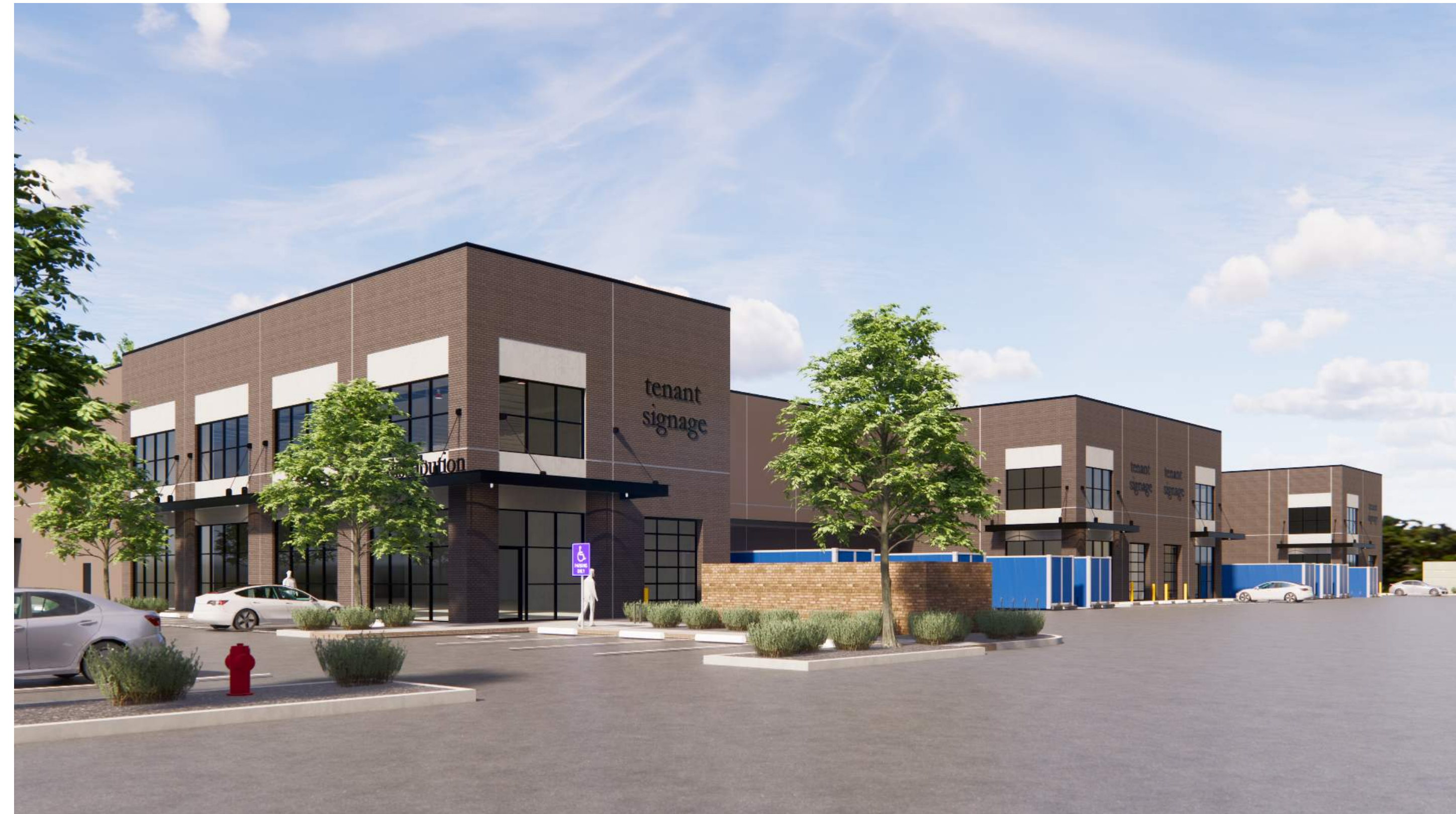
BUILDING 3 - NORTHWEST ELEVATION
